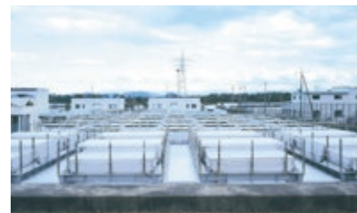
Yoshikawa water purification plant (Shiga Prefecture)
