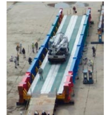
Temporary bridge for use in emergencies (Kinki Regional Development Bureau, Ministry of Land, Infrastructure and Tourism)
