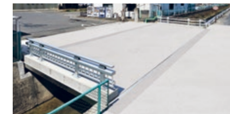
Bridge with aluminum plate deck (in the premises of Kambara Complex of Nippon Light Metal Co., Ltd.) Many large vehicles cross this bridge for shipments and deliveries.
